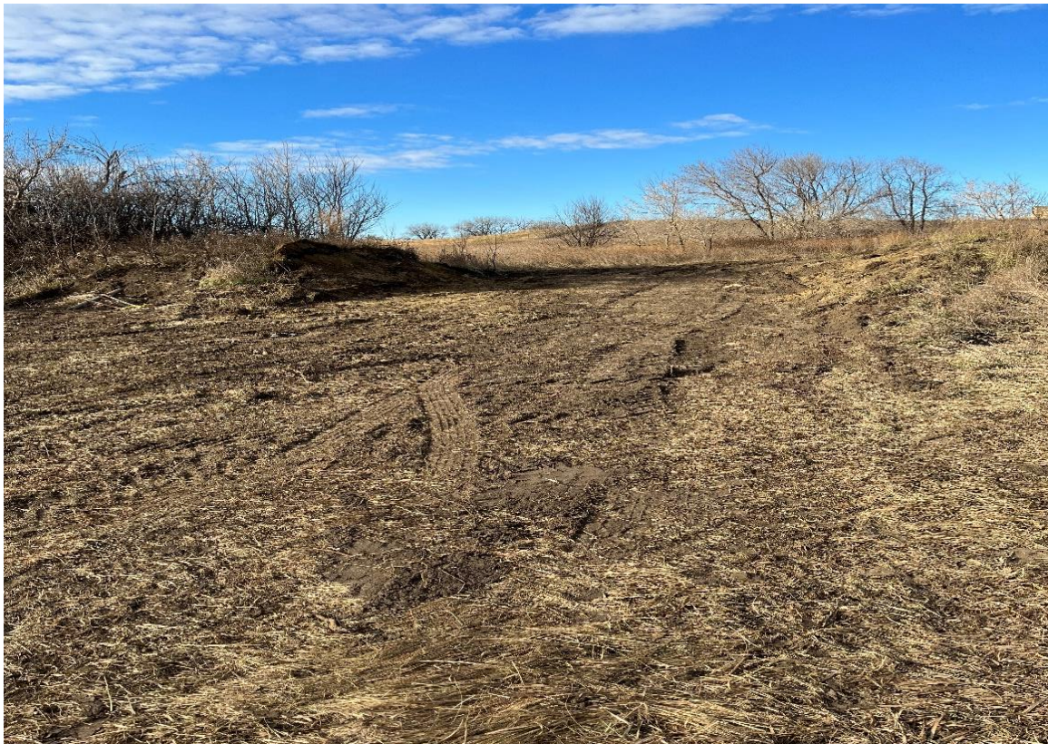
Figure 5: The borrow area after it was graded and seeded.
